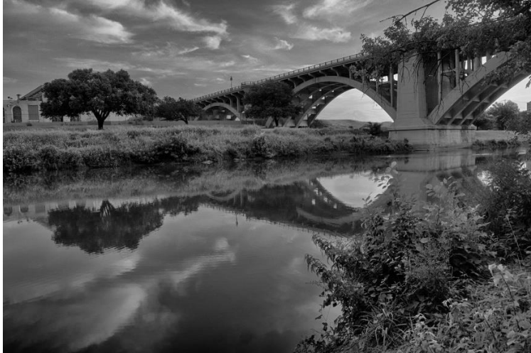
Main St Bridge from Trinity Trail
